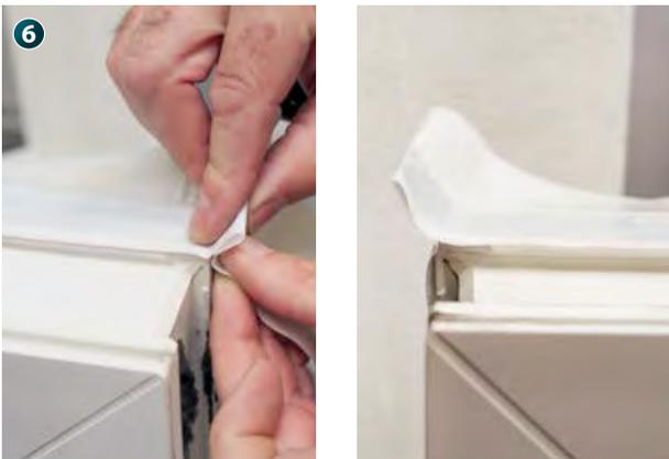
Add a loop at each corner with the size of the respective joint dimension.
