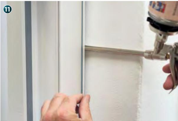
The joints can now be almost completely filled with a suitable insulating material.
