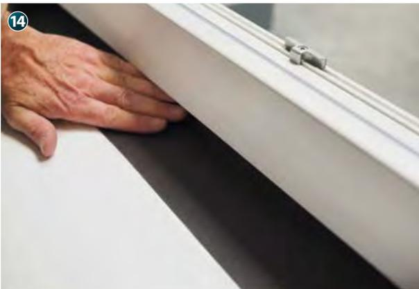
When attaching the tape to the building structure, make sure to leave a pronounced trough.
