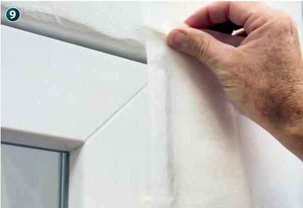
With the moisture-variable Hanno®-Flashing Tapes you can seal both the internal and the external connection. Alternatively special Hanno®-Flashing Tapes for exterior respectively interior applications can be used.
