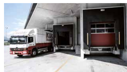
Installations de quais
