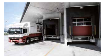
Installations de quais
